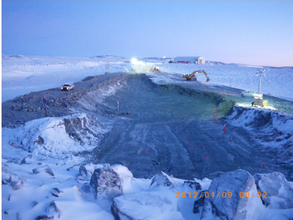
Photo 3: Current conditions of the base of the key trench.
