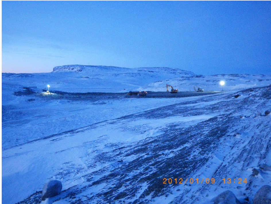
Photo 1: Removal of the ROQ protective cover from the upstream side of the key trench. The ROQ was placed along the upstream face of the dam.
